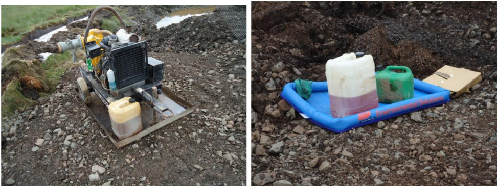
Plate 12: Examples of drip trays and bunds
