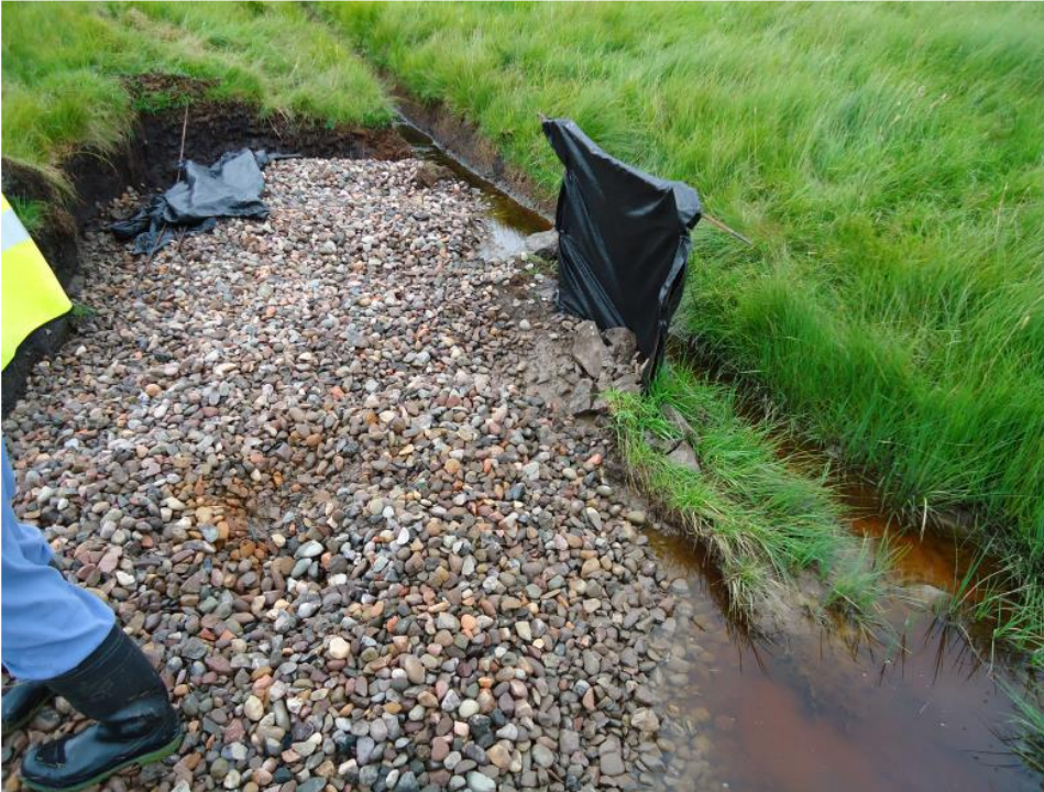
Plate 2: Typical silt traps
