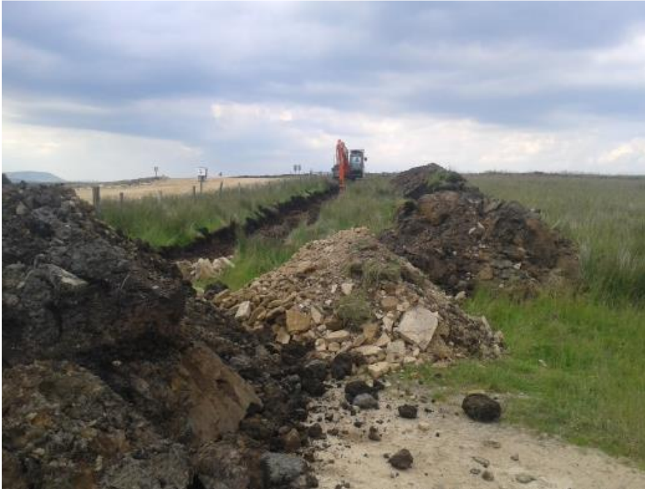
Plate 14: Typical overburden stockpile measures
