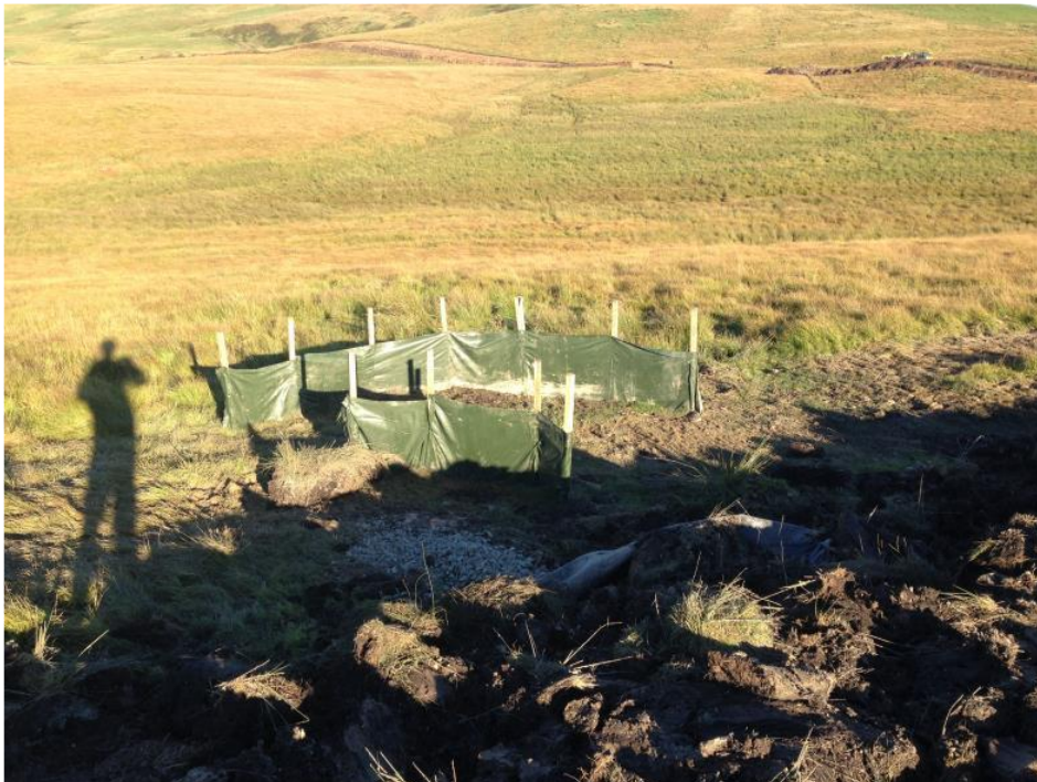
Plate 1: Typical silt fencing
