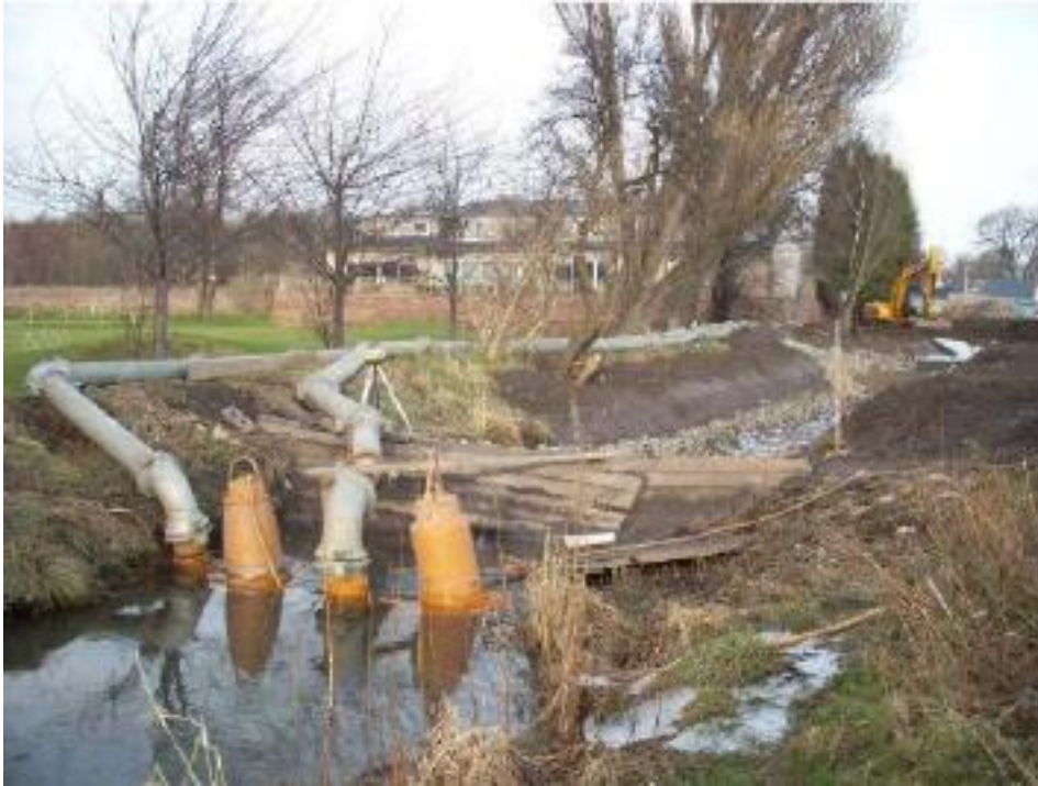
Plate 8: Full isolation - over pumping/siphon
